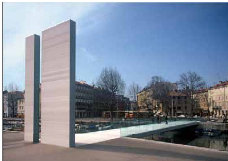
MEMORIAL BRIDGE / RIJEKA / 3LDH / 2005
